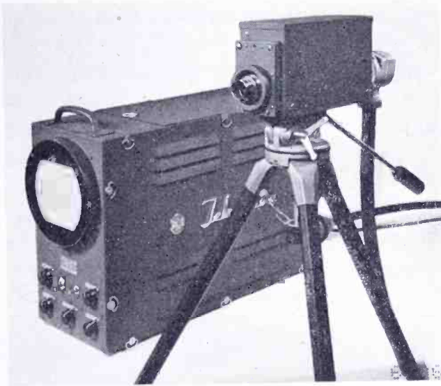
Miniature television camera employing the vidicon pickup tube 6 , monitor in background.
